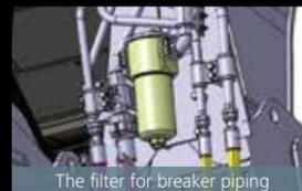
The filter for breaker piping
